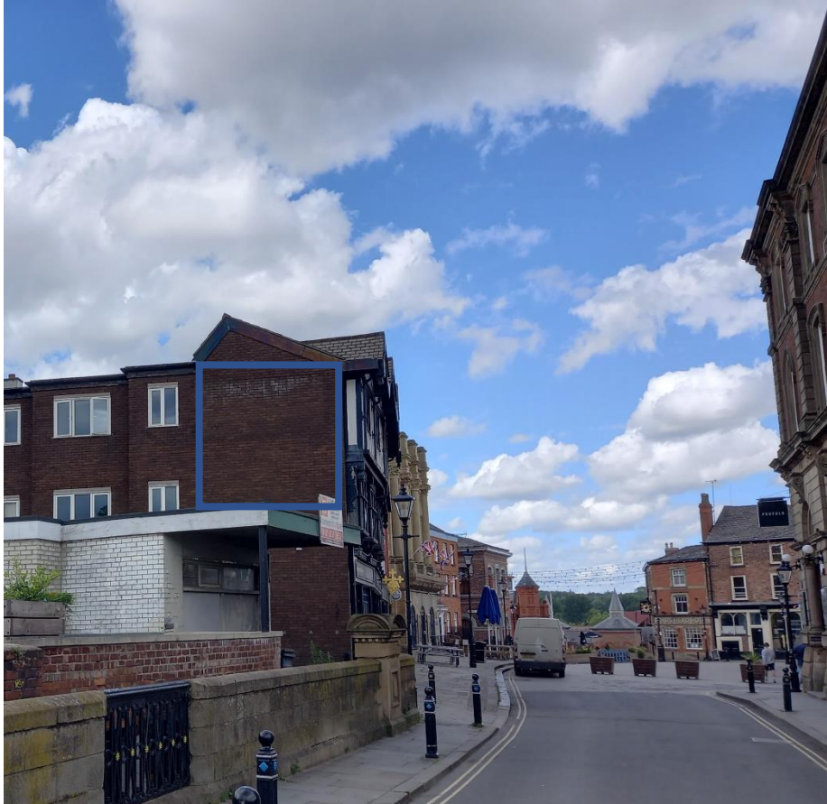
18-19 Marketplace (surface: brick, can be seen from St Petersgate Bridge)
